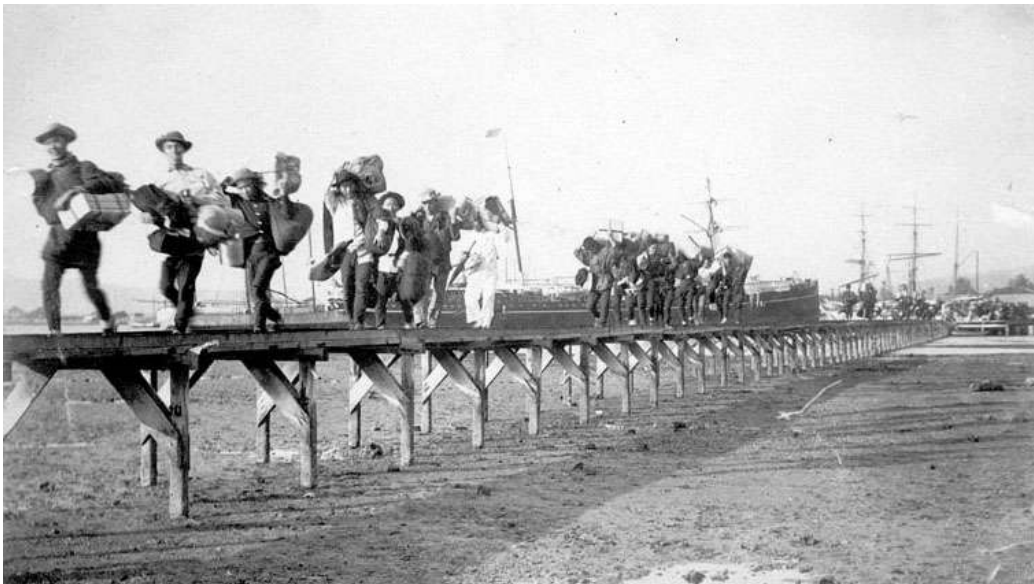
Half-mile long wooden bridge connecting the harbor and Quarantine Island
